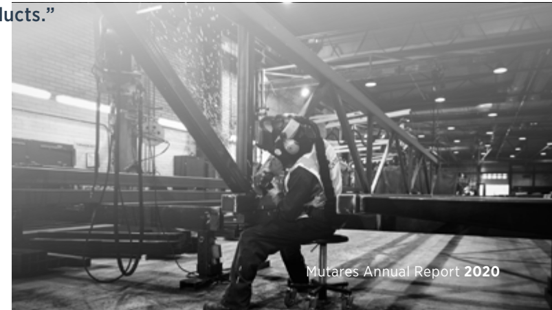
Manufacturing parts for a highway bridge
