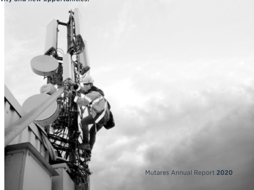
Employee during maintenance on site
